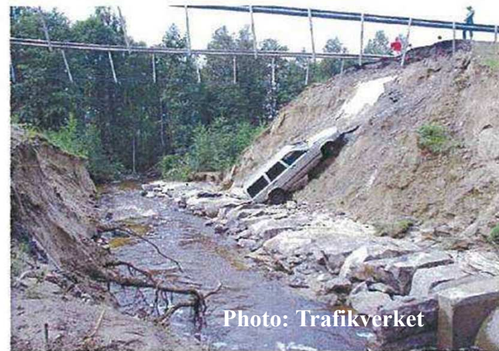
Erosion, Road 240, Hagfors
